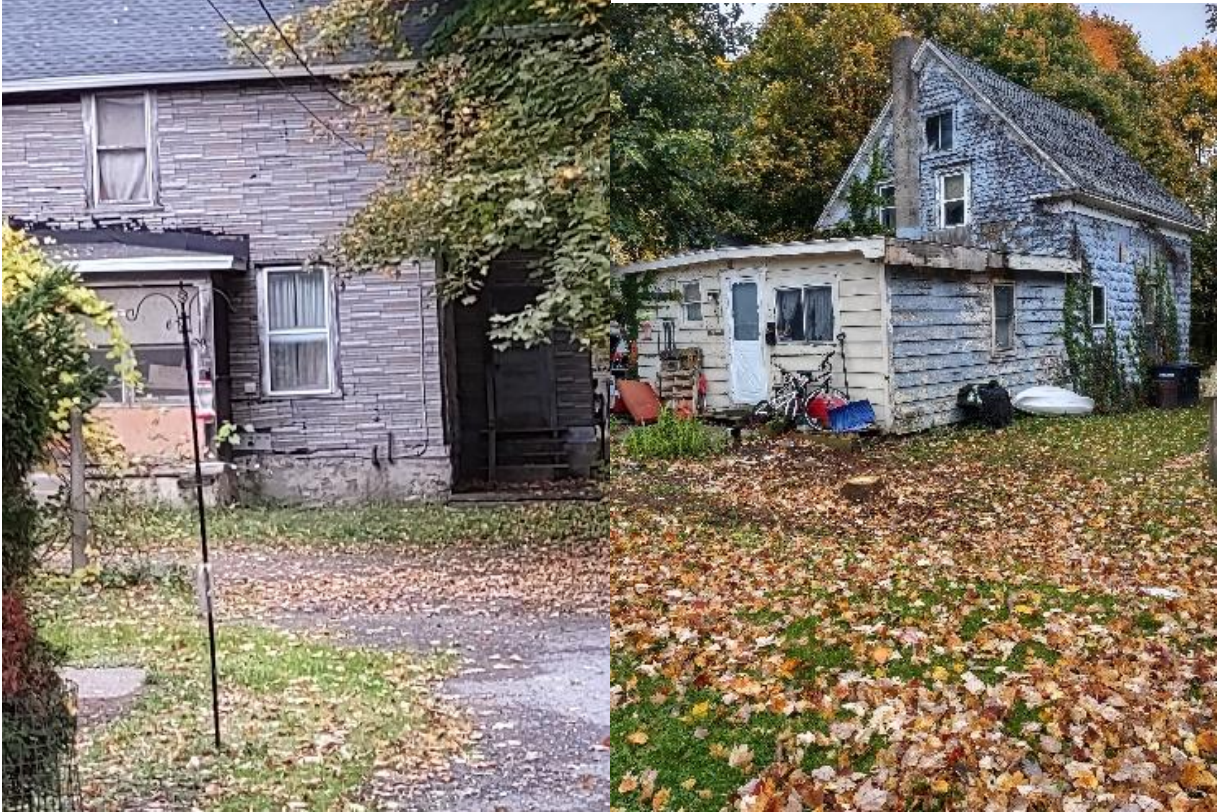
Hunt St. (behind the post office)
